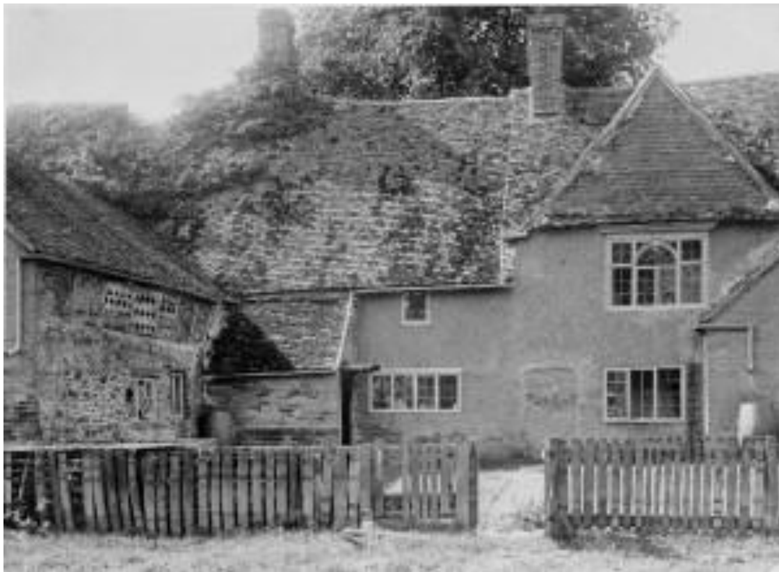
Photo of old house at Lime Close
